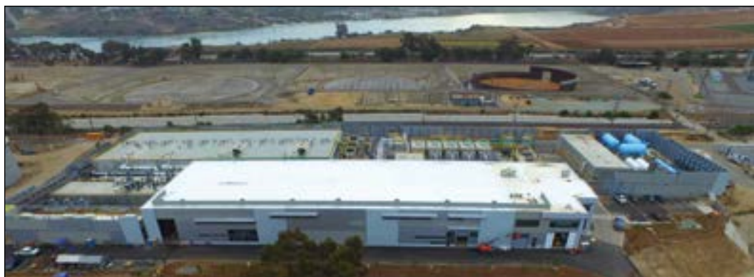
The Carlsbad Desalination Plant will be commissioned in late 2015. Photo courtesy of Poseidon Water
