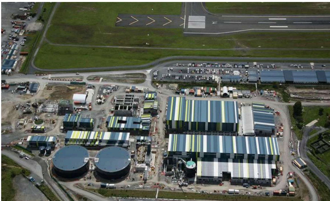
Figure 10 – Gold Coast Seawater Desalination Plant Source: WaterSecure
