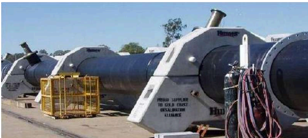
Figure 6 – Outfall with Diffusers - Gold Coast Desalination Plant, Australia Source: The Water Corporation
