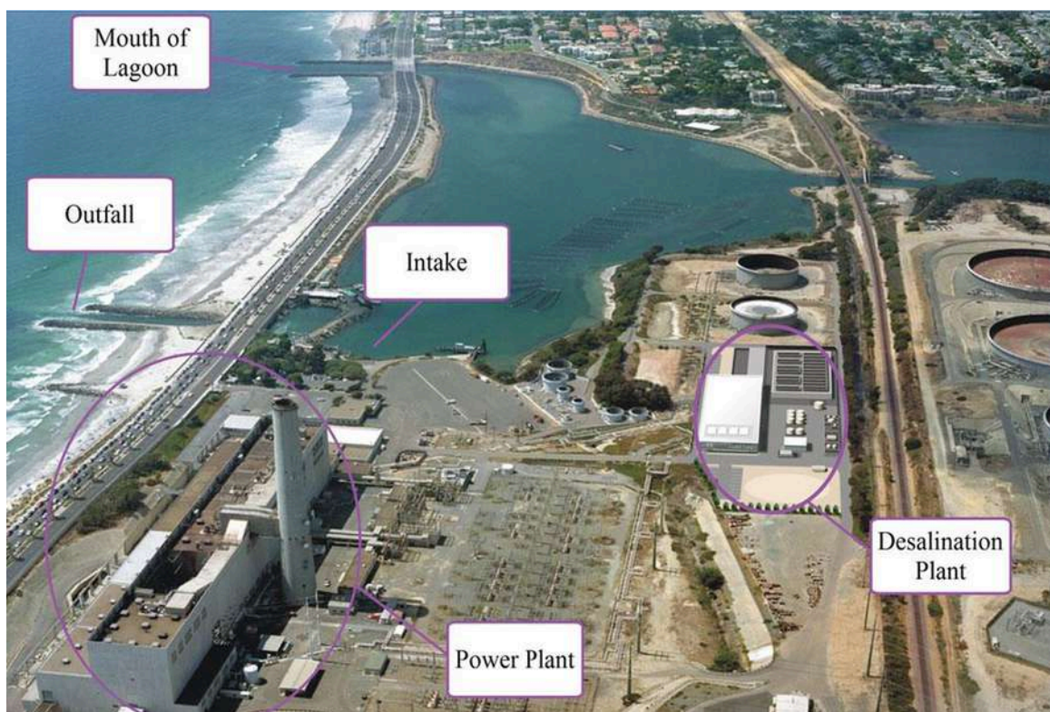
Figure 3 – Carlsbad Desalination Plant Near-shore Discharge Source: Poseidon Water
