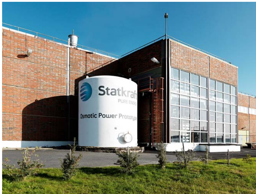
Figure 9: Prototype osmotic power plant, Tofte, Norway. (Photo: Damian Heinisch / Statkraft).
